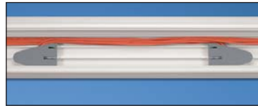
TGFSB installed in TG-70 Raceway
